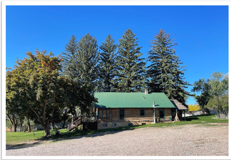
Figure 9: Existing Ranch House at 4000 CR 115
